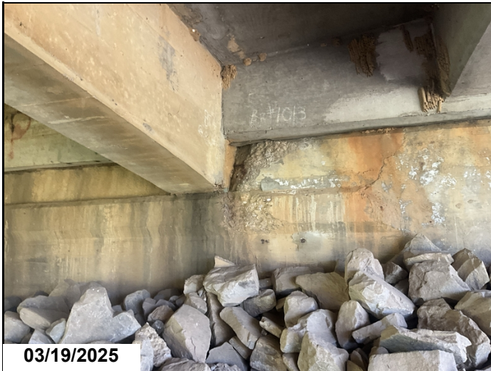
Abutment #2, girder # 4: spalling with exposed reinforcing steel adjacent to girder # 4.
