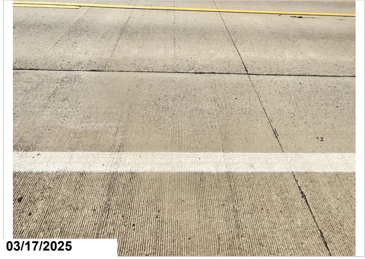
Sealable deck cracking.
