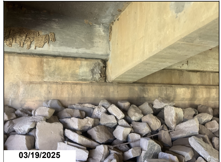
Abutment # 1, girder # 4: spalling with exposed reinforcing steel adjacent to girder # 4.
