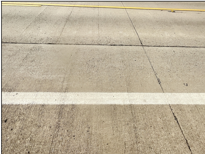
Sealable deck cracking.
