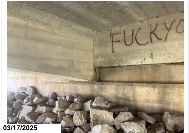
Abutment # 1, girder # 4: spalling with exposed reinforcing steel.
