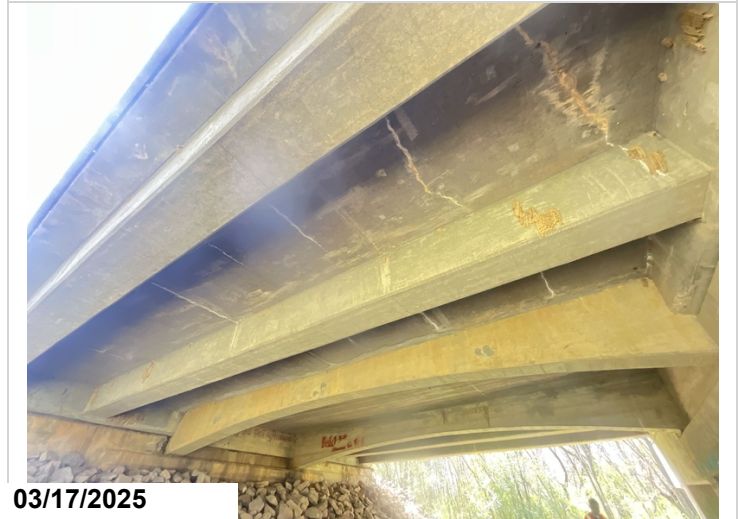
Undersurface, Span # 1: typical.
