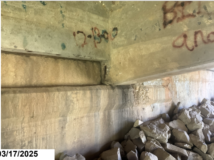
Abutment # 2, girder # 4: spalling with exposed reinforcing steel.
