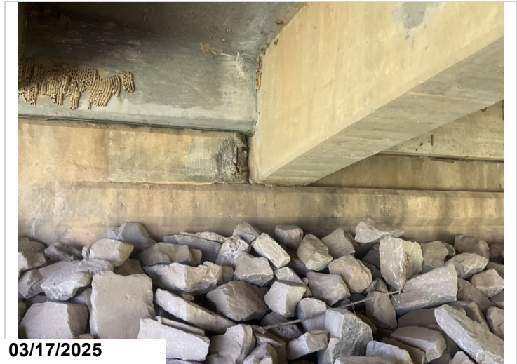
Abutment # 1, girder # 4: spalling with exposed reinforcing steel adjacent to girder # 4.
